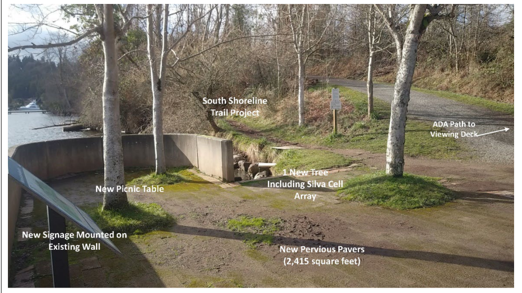
Diagram 5 Locations of New Pervious Pavers and Silva Cell at South End of Plaza (Looking South)
